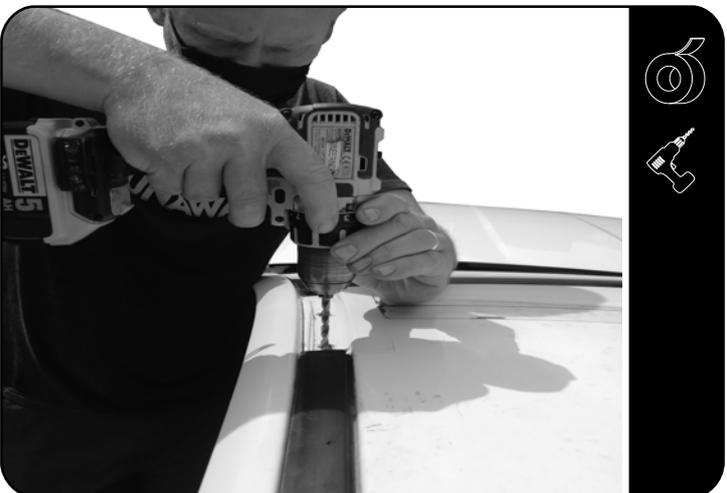
Drill the 6 holes you marked earlier, starting with a 4mm pilot hole before widening to a 7mm hole. There is no need for a lot of downward pressure. Let the drill do the work.
